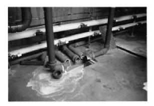
Note 1—Floor drains come in various shapes and sizes. Shown here is one type of floor drain. It is important to know the point of discharge of any floor drain.
