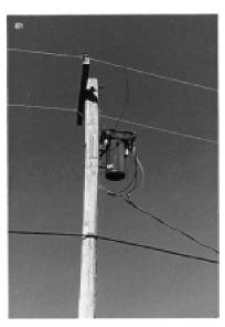
FIG. X2.3 Typical Pole-Mounted Transformer
