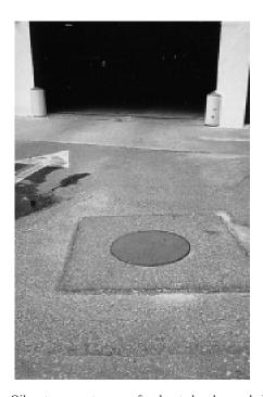
Note 1—Oil-water separators are often located under manholes outside repair garages, or at any location where it is necessary to separate oil from water prior to discharge.
